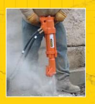
A general rule of thumb when sizing the appropriate breaker for your application is to use 10 pounds for each inch of material. A 40-pound breaker, for instance, is a good fit for 4-inch concrete. A 90-lb breaker would be used to break 9-inch concrete.
